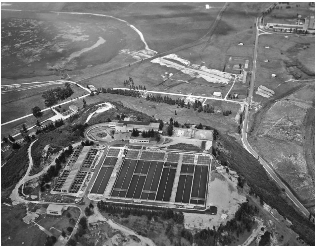
Saúl Ordúz, Tibitoc Treatment Plant , 1974
