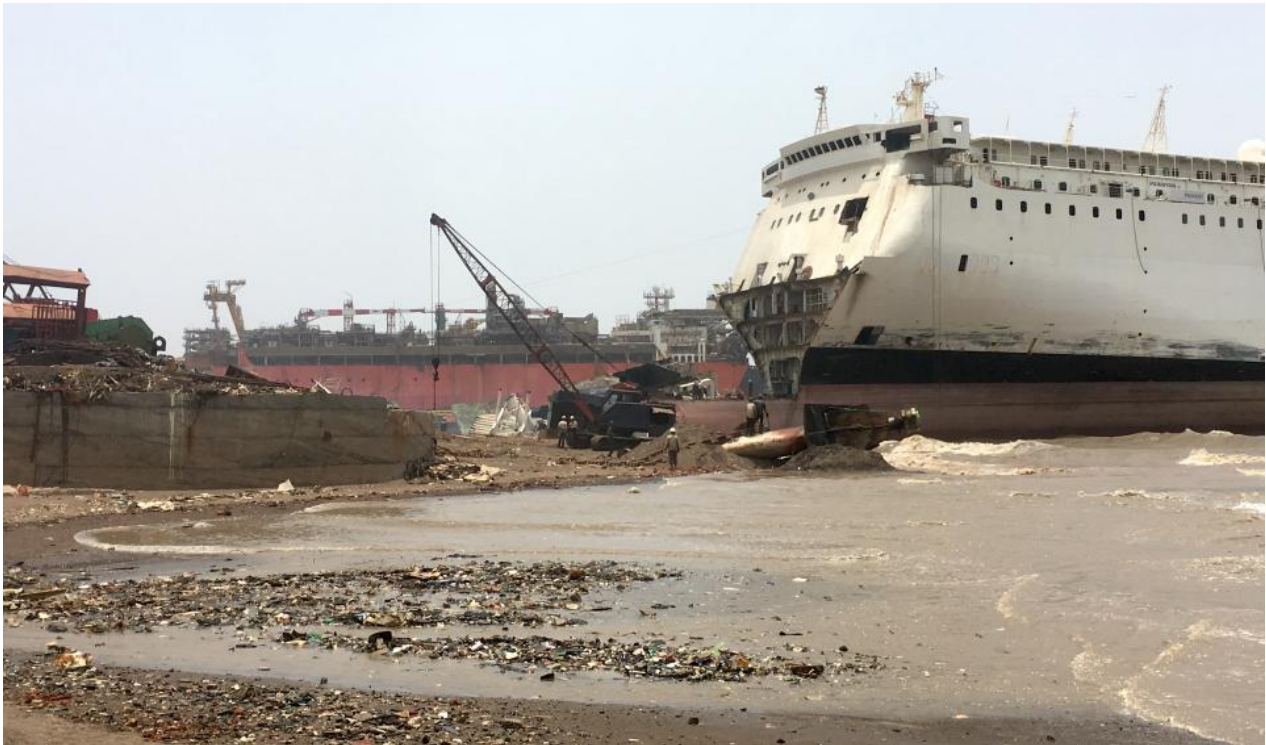
Shipbreaking in progress, with a cut being made on the nose of the ship in Alang, Gujarat. Photograph by Ayushi Dhawan, 2018.
